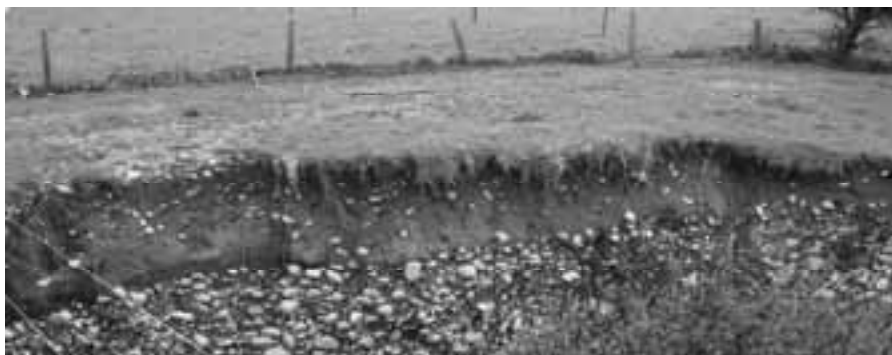
Plate 79: Moderate streambank erosion exposing stony Kopua soils in the Tararua district. Gravels at 45 cm (LUC 3s) and an appreciable size and number of stones occur in the profile and often at the surface (stone picking is common). Also note the slight depression (1D) of fine gravels from a previous flooding event (AKM).
